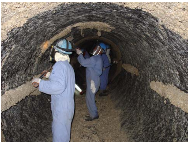
Removing marine growth and the old dosing line and anodes
