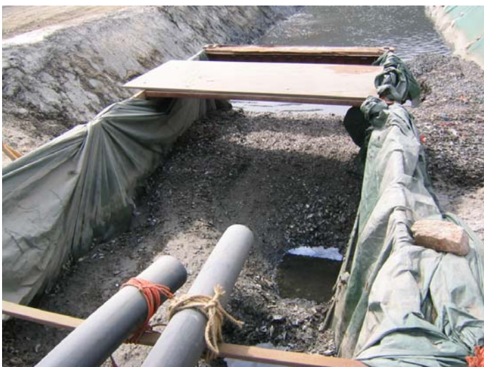
Drying of the debris slurry prior to removal
