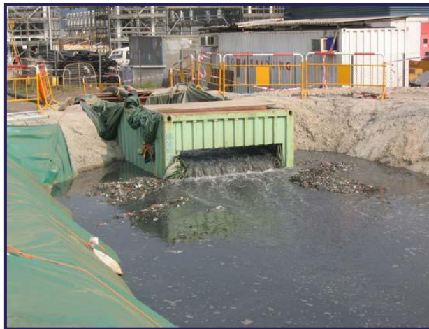
Collection of debris slurry into temporary stilling basin
