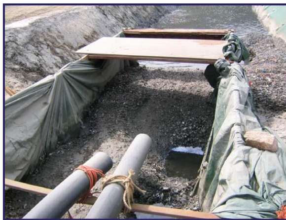
Drying of the debris slurry prior to removal
